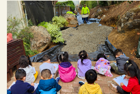
2023: Pre-K visits the construction daily to draw the changing space and ask the builders questions.
